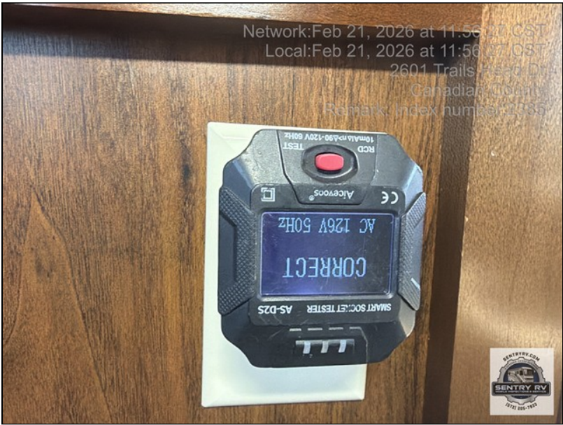
Voltage/Polarity/Frequency Test Kitchen Counter
