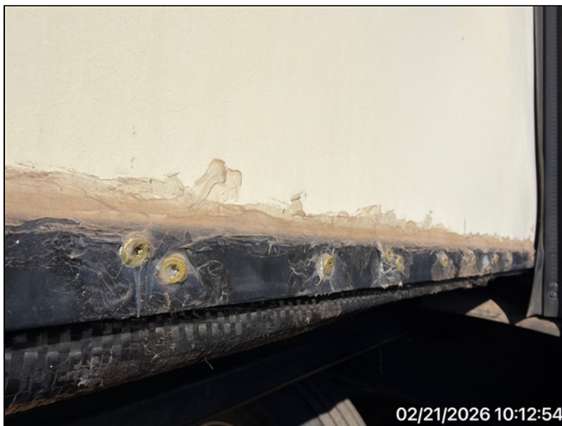
Curbside Slideout Lower Front Repairs
