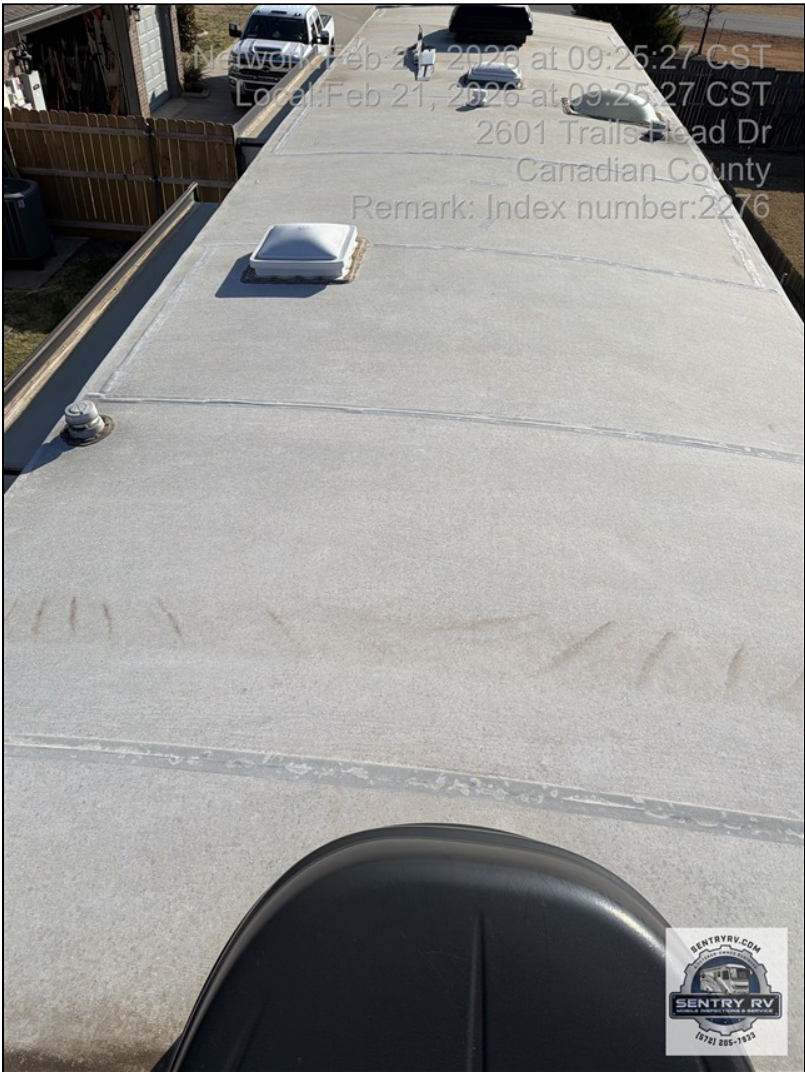
Roof Back to Front
