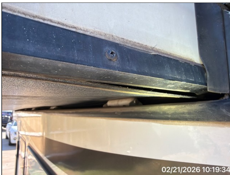
Streetside Front Slideout Floor
