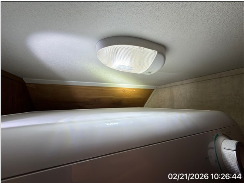
Ceiling Above Washer/Dryer
