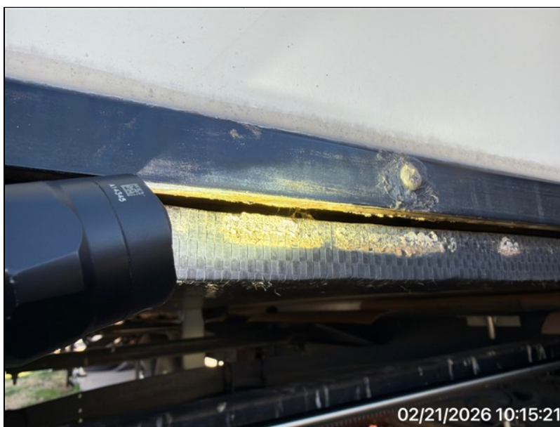
Streetside Rear Slideout Wall/Floor Junction
