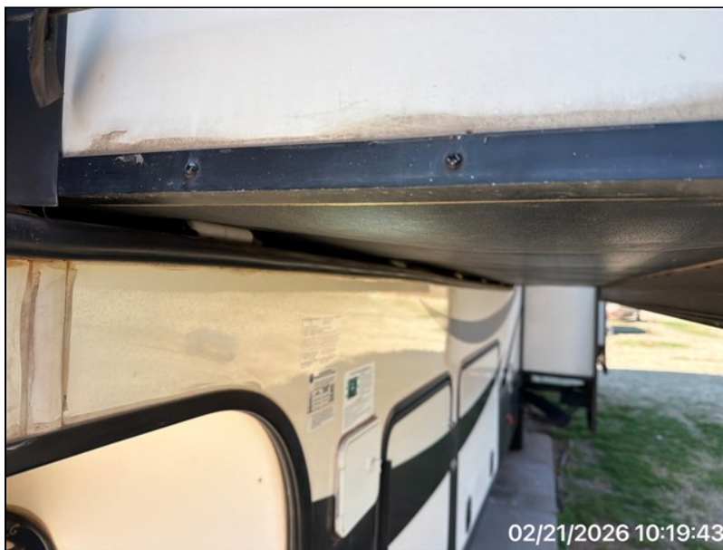
Streetside Front Slideout Floor
